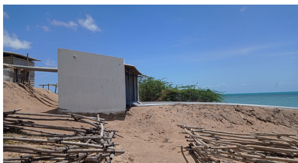
An aquafarm motor room within the high tide line, which is against the Coastal Aquaculture Authority regulations (Photo: Prabhakar Jayaprakash)
